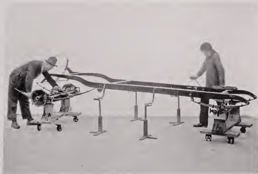
OPERATION NO. 1 Assembling Model 250
